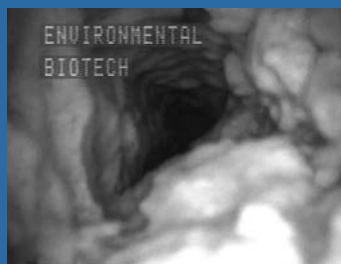
Urinal 2 – before: 70-80% restricted with large build-up.
